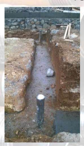
Ground beams will directly be inserted and poured on the piles cap.
